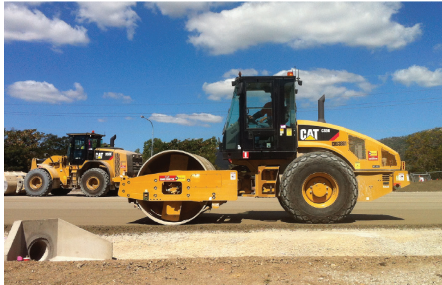
FIGURE 1.2 Soil compaction for a highway construction project (Courtesy of N. Sivakugan, James Cook University, Australia)
