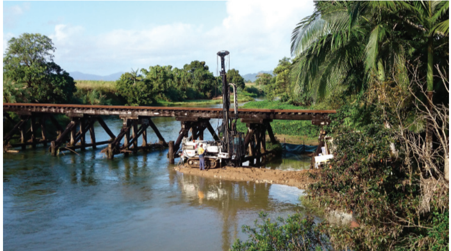
FIGURE 1.1 Soil exploration program (Courtesy of N. Sivakugan, James Cook University, Australia)
